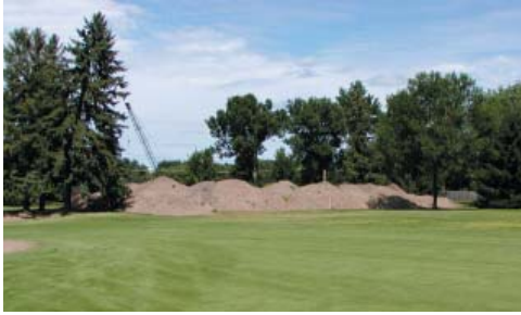
Soil stockpiled at the proposed hole 12 green site.
