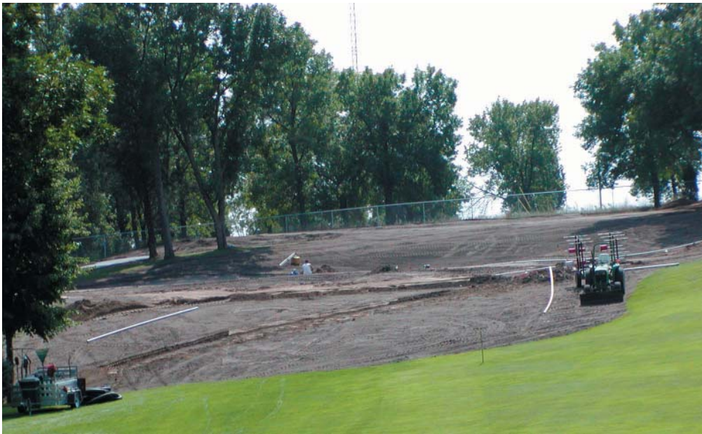
Early in the construction process at the hole 14 green site.
